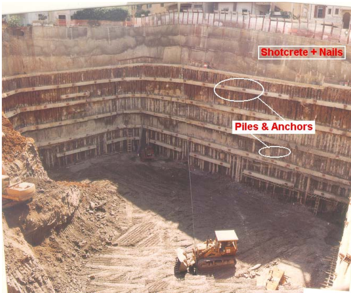
Fig 7. Temporary Shoring of a Deep Excavation
