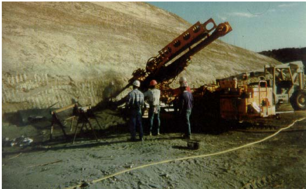
Fig 8. Slope Stabilization with Permanent Anchors
