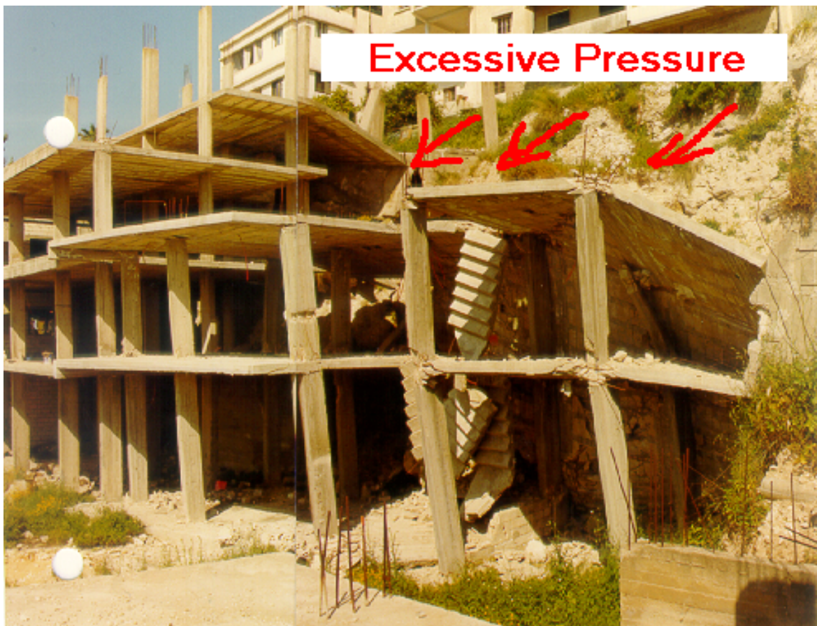
Fig. 3. Failure of a Building Skeleton due to Excessive Lateral Pressure
