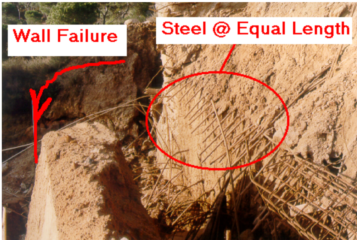
Fig. 5. Total Collapse of a Cantilever Wall due to Steel Congestion and Pull out, With Foundation on Unyielding Piles and Poor Drainage
